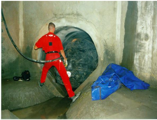
7. Fill the Conical Plug until the material will lay around the pipe wall without any pressure.
