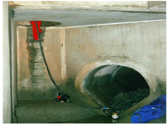
8. Leave the manhole! Pressurization with the full working pressure of 1 bar must be carried out from outside the manhole.
